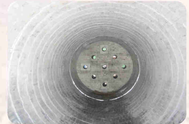
Carbon Black reactor after repair / lined with corundum special bricks LUPUDUR K 99
