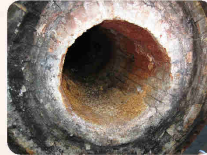
Carbon Black reactor before repair
